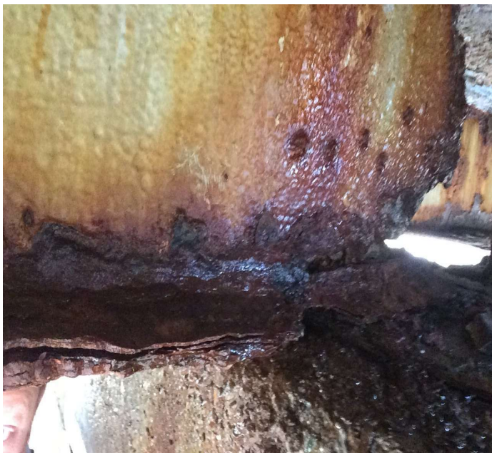
PHOTO 4 Description Girder 2 at Beginning of Span 2 has severe section loss to bottom of web and bottom flange with large hole in bottom of web and is beginning to crush.
