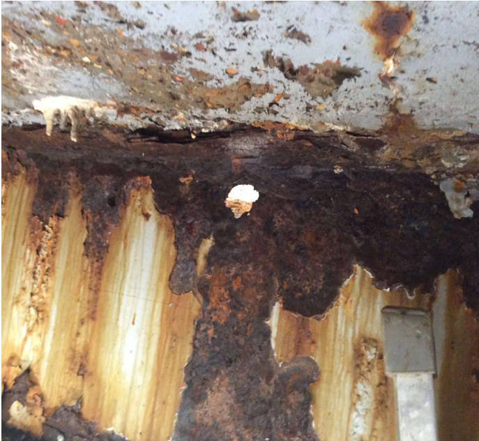
PHOTO 7 Description Girder 3 has hole in top of web near 1/4 point @ Span 2.
