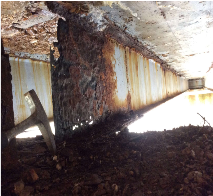
PHOTO 8 Description Girder 10 at End of Span 1 has severe section loss to end of web with hole at end of Girder.
