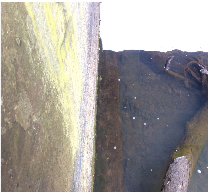
PHOTO 1 Description Scoured 1' below top of footing @ Bent 1.
