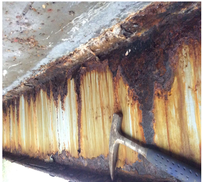
PHOTO 6 Description Girder 3 has hole in top of web near midspan @ Span 2.
