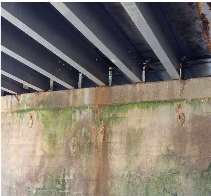
PHOTO 1 Description Spalls to Cap on ahead side of Bent 1.
