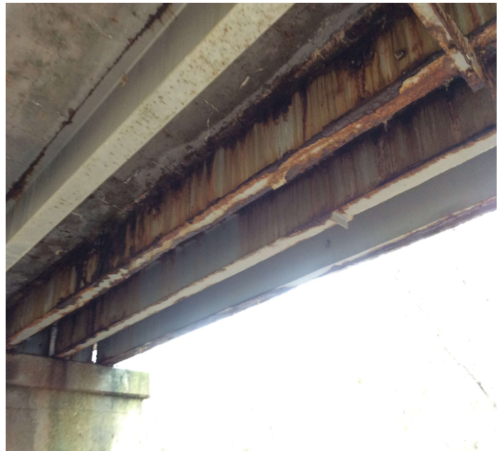
PHOTO 5 Description Rust & section loss to Girders 1 - 3 @ Span 2.
