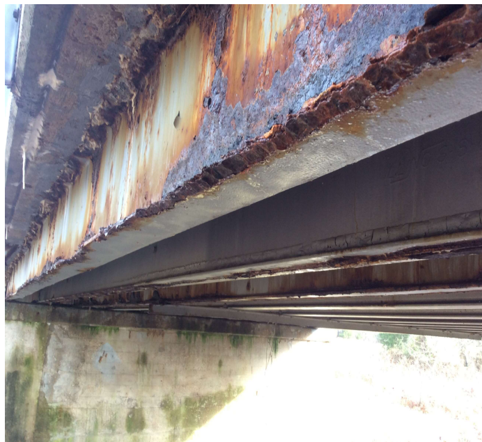
PHOTO 1 Description Rust & section loss to Girders 1 - 3 @ Span 1.
