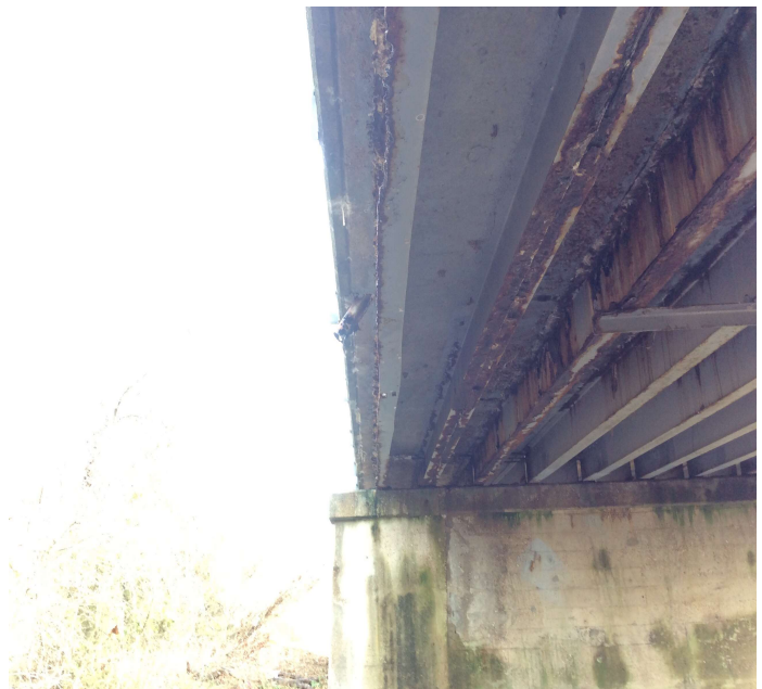
PHOTO 2 Description Distortion to Girder 1 @ Span 1.
